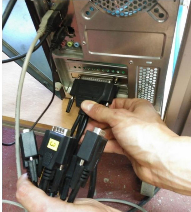
Figure 85: Connection between the PC and the network analyzers t
